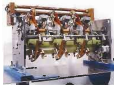
Converted GE LRT200-2 Load Tap Changer
